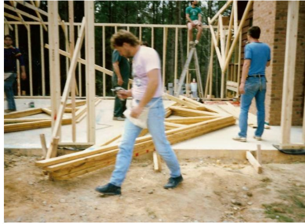
Jim building a garage in NC
